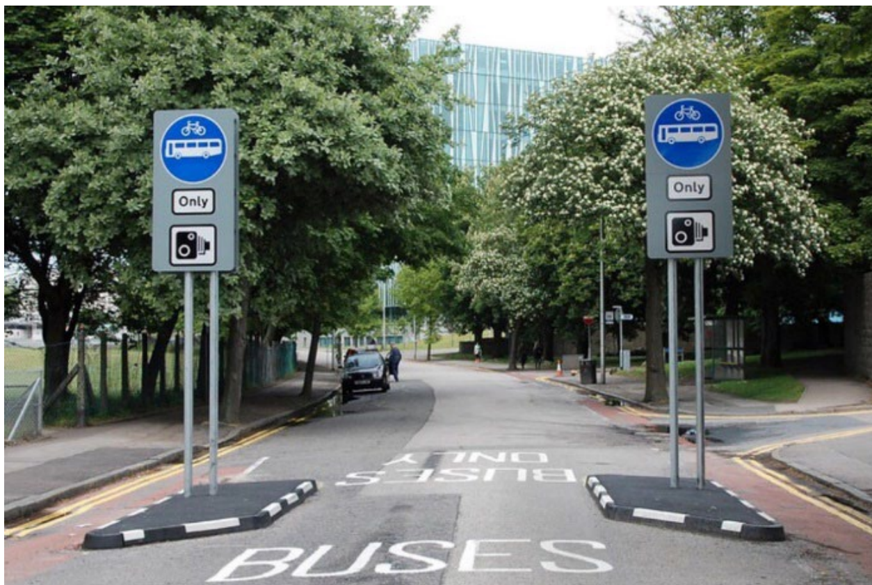
(Figure 23: bus gate with cycling permitted and camera enforcement)
