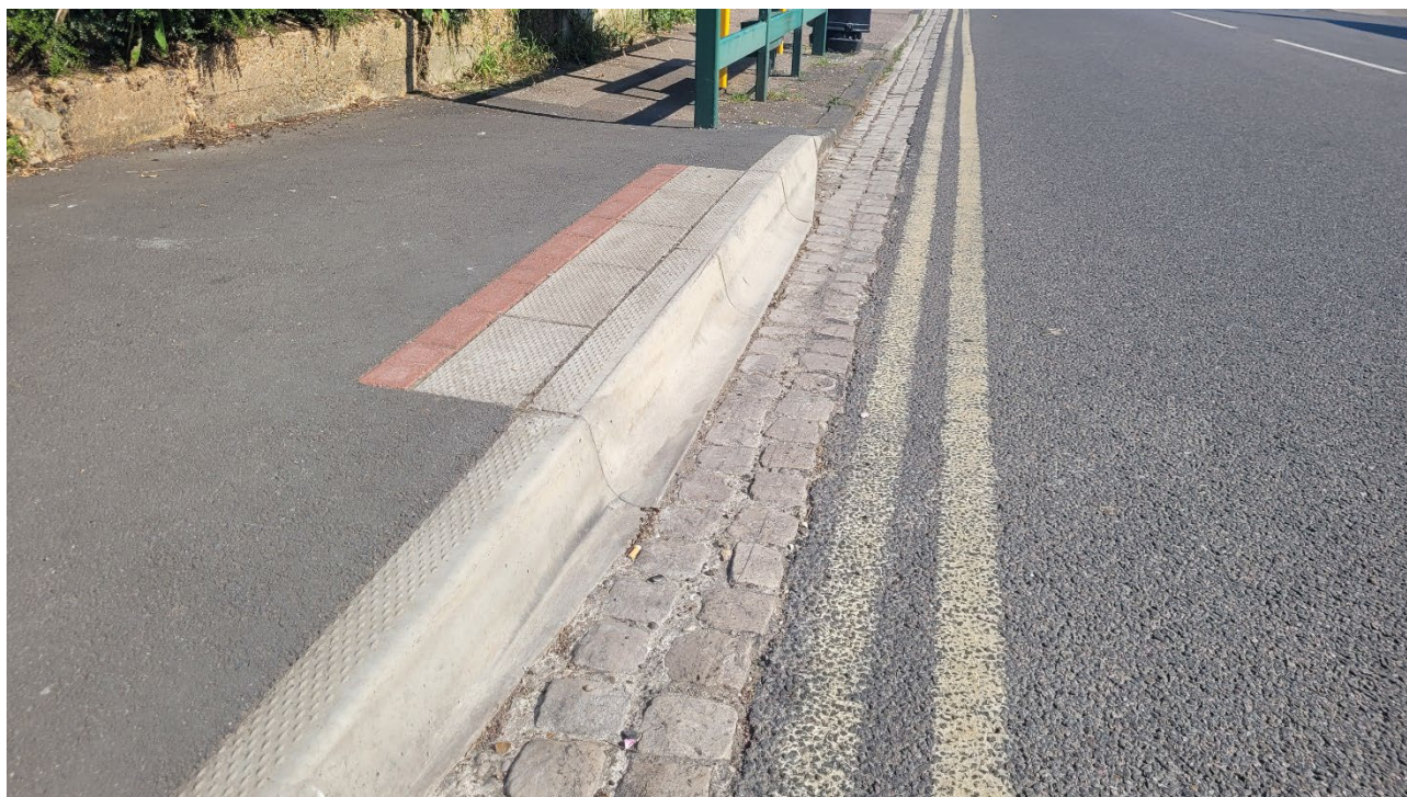
(Figure 7: raised kerb for ease of boarding and alighting)
