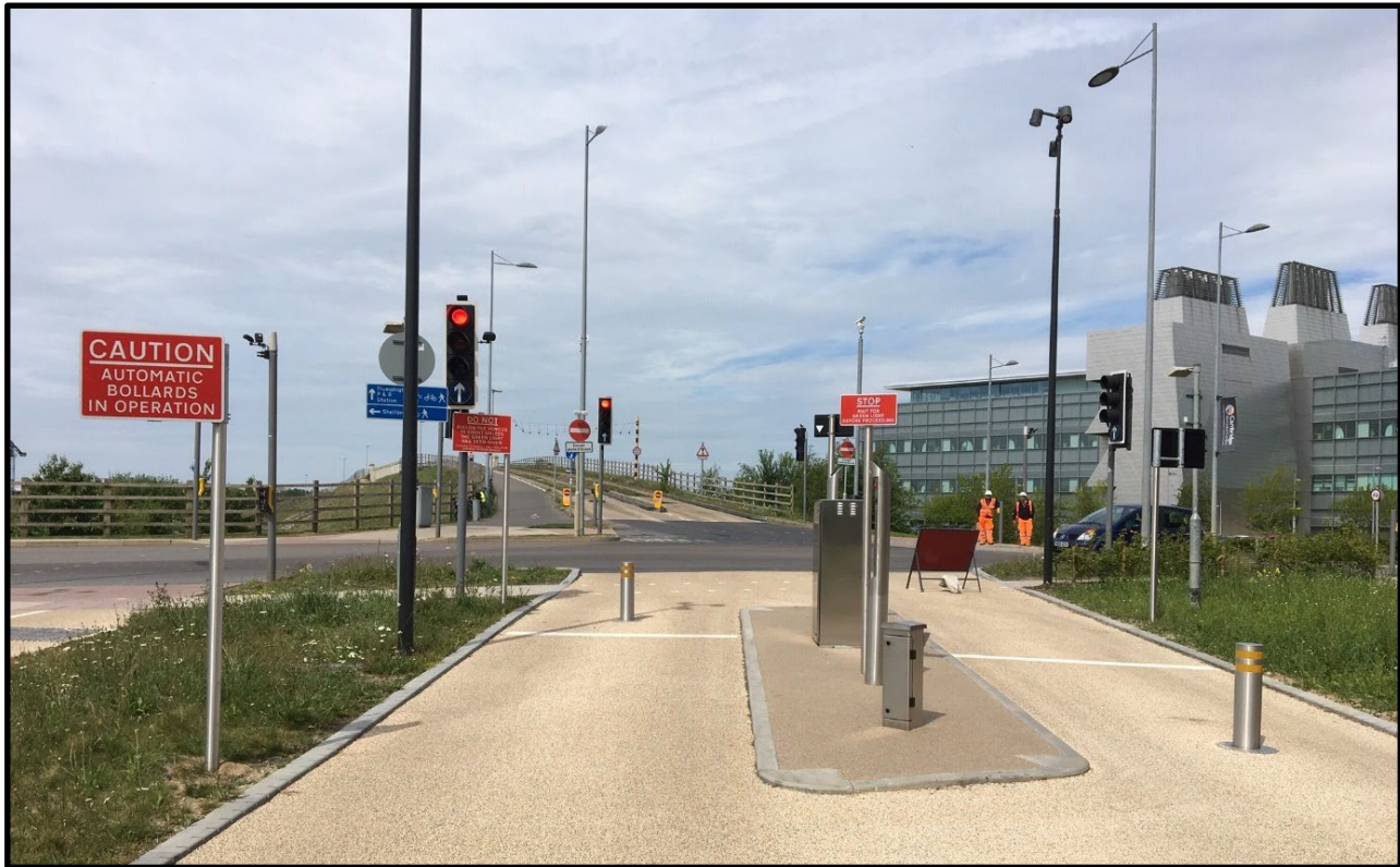
(Figure 32: TSP with integrated bus bollards and AI camera)
